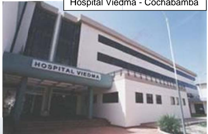
Hospital Viedma - Cochabamba
