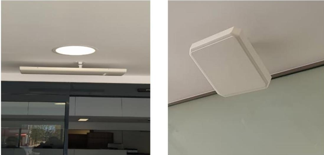
**Figura 12.** Antena lector RFID RFMAX S9028PCR
