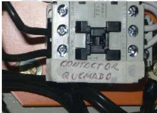
*Figura 3.5 Contactor Quemado*
