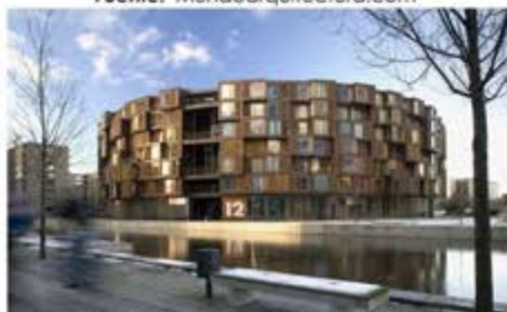
Fig.30 Vista Exterior Tietgen Student Hall Fuente: Tietgen Student Hall
