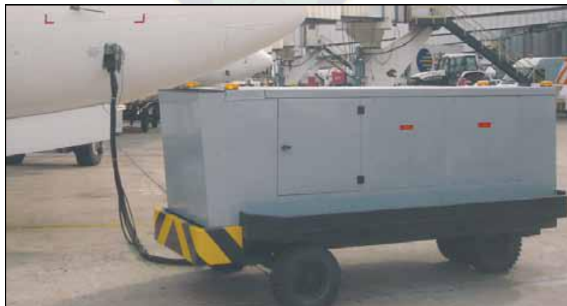
Figura 6.3 Ground Power Unit (GPU)
